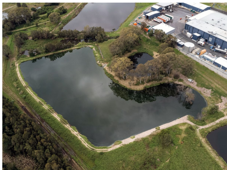
Primary processing facility, Queensland
